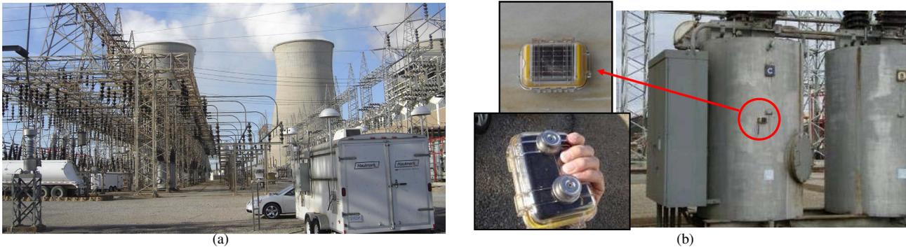
Fig. 1. (a) View of the Paradise substation, where the *ParadiseNet* was deployed. (b) One of the wireless sensor nodes for circuit-breaker monitoring.
