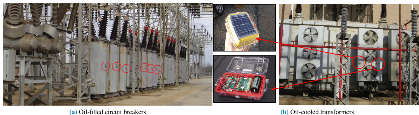
FIGURE 3: Illustrations of wireless sensor nodes deployed in ParadiseNet : (a) locations of surface temperature sensor nodes, and (b) temperature, vibration, and sound intensity sensor nodes.
